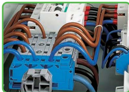
Rail-mounted distribution terminal block with 35 mm<sup>2</sup>/AWG 35 screw clamp connection (front-entry) and 3 x 10 mm<sup>2</sup>/AWG 8 front-entry CAGE CLAMP® connection.
