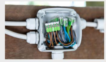
The Green Range Splicing Connector with Levers can be used for wiring in distribution boxes – like here, at a charging station for e-bikes.
