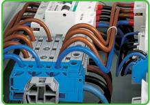
Rail-mounted distribution terminal block with 35 mm²/AWG 35 screw clamp connection (front-entry) and 3 x 10 mm²/AWG 8 front-entry CAGE CLAMP® connection.
