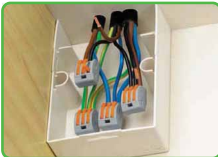
Connecting pre-wired and pre-fabricated components; e.g., modular assemblies used in mobile homes.
