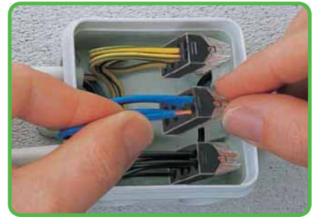
Termination: Insert stripped, solid conductor fully.
