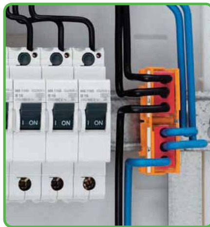
Terminating solid and stranded 6 mm 2 /AWG 10 conductors.
