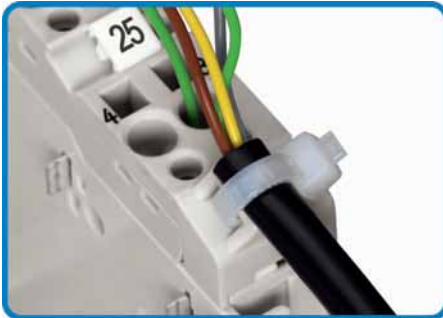
Securing the cable on the connector
