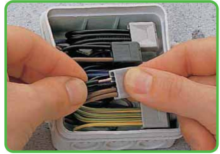
Termination: Insert stripped solid conductor fully.
